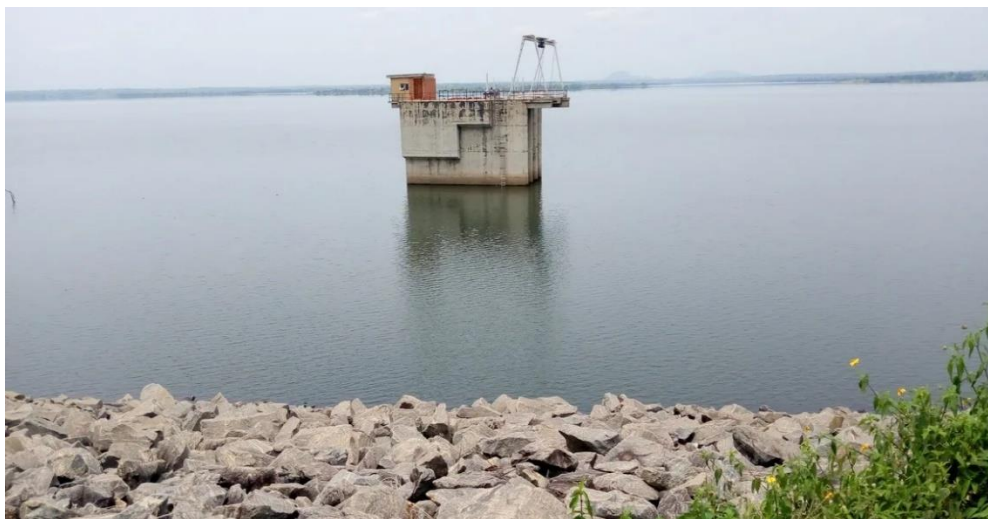
Figure 2. The Ikpoba dam
